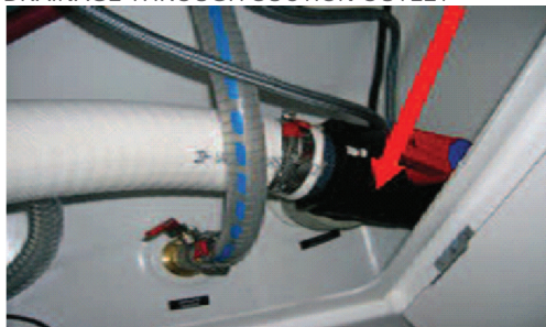
DRAINAGE THROUGH SUCTION OUTLET -
